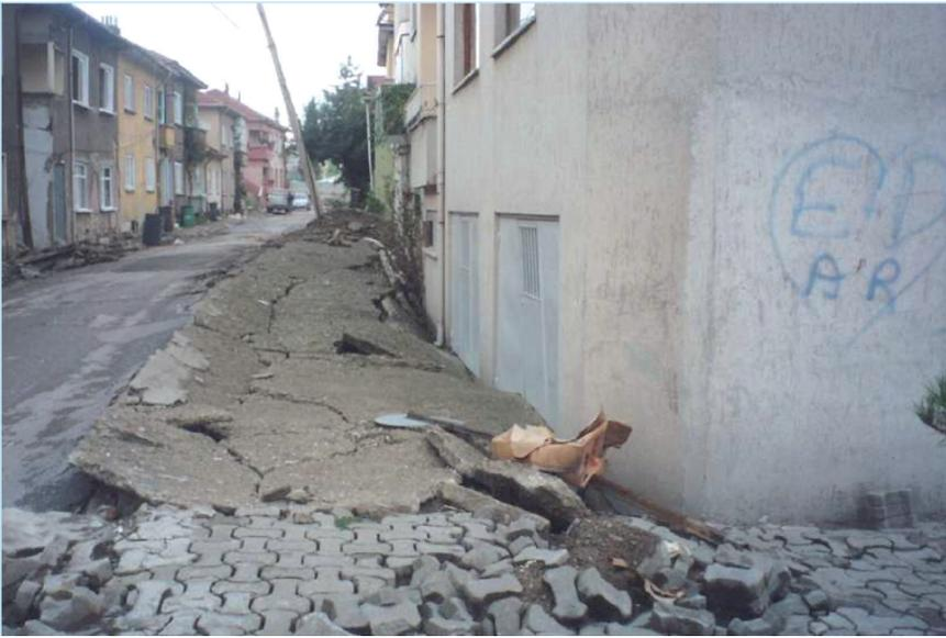
Figure 1.1- 3 – Effects due to liquefaction (Izmit, Turkey, 1999).
